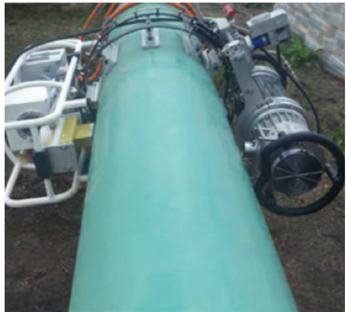
Fig 1. Portable Real Time Radiographic unit for pipeline inspection. Courtesy Shaw Pipeline Services.
